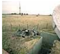
Remains of supporting girder framework
